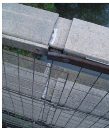
Photo 7.3 Parapet expansion joint
