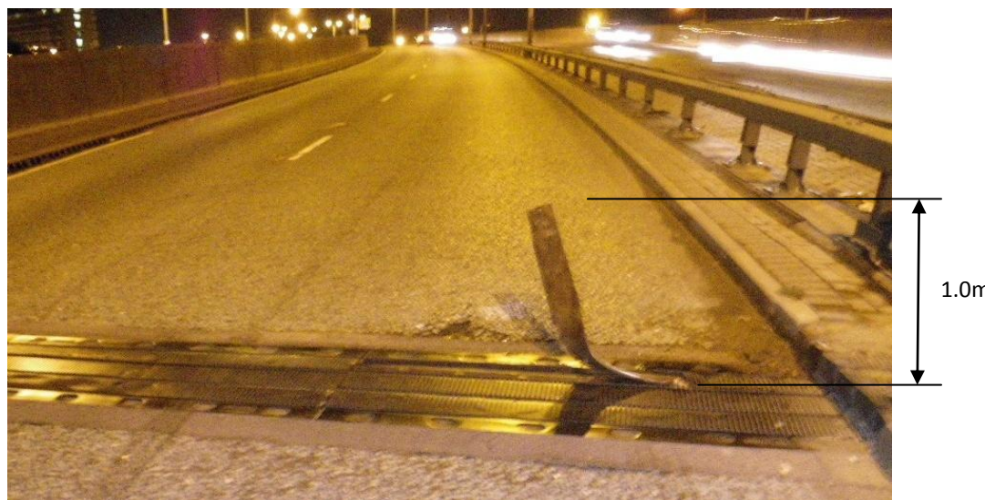
Photo 2.1 Failed elastomeric expansion joint on a major dual carriageway
