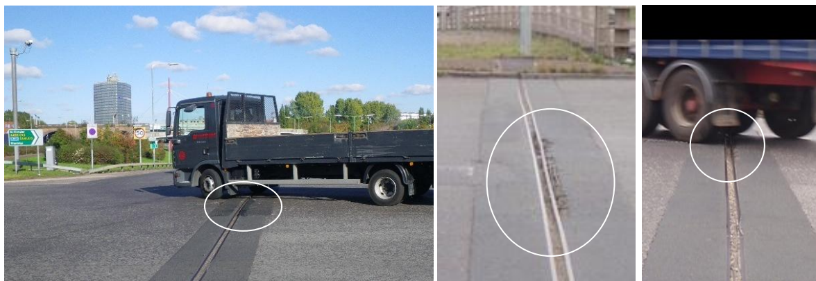
Photo 7.5 Expansion joint at a turning point
