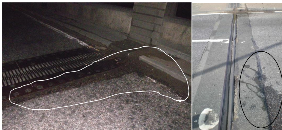
Photo 5.4 In both examples, the carriageway is wet on one side of the joint, showing that the surfacing is saturated.
