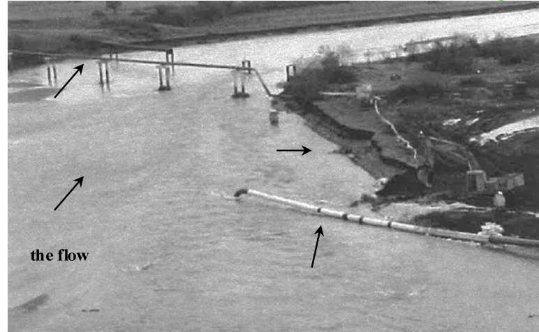
Scour at pipelines
