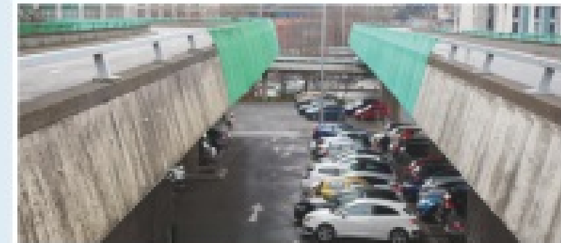
Green netting on parapets protects cars from falling material
