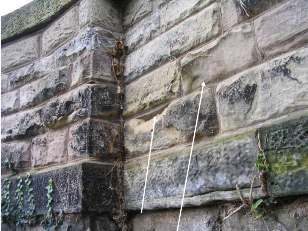
Photograph 2C.19: Example of a stone wing wall where the depth of the defect \geq 20\text{mm} (Severity rating D)
