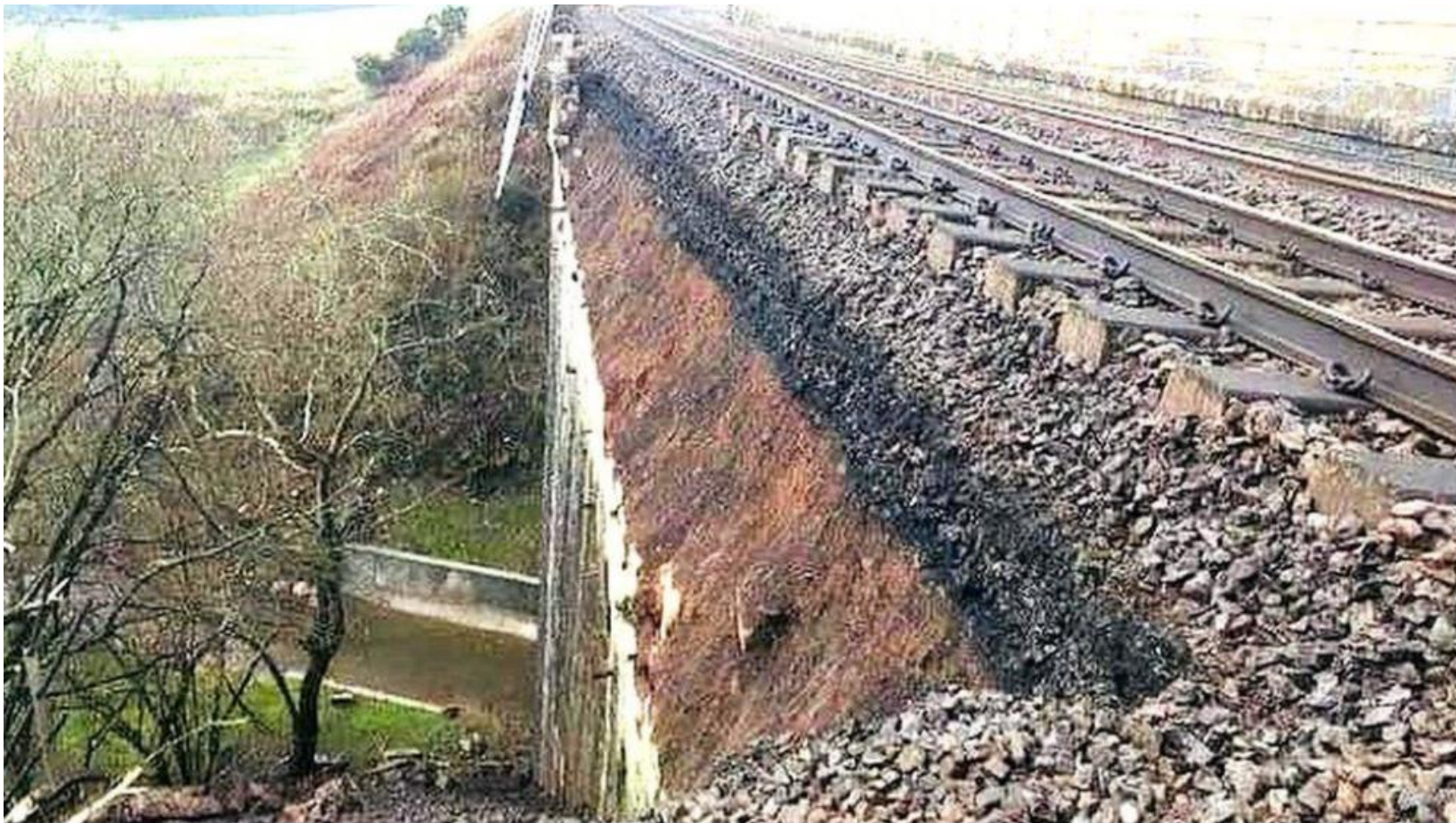
A 24m section of the bridge parapet collapsed
