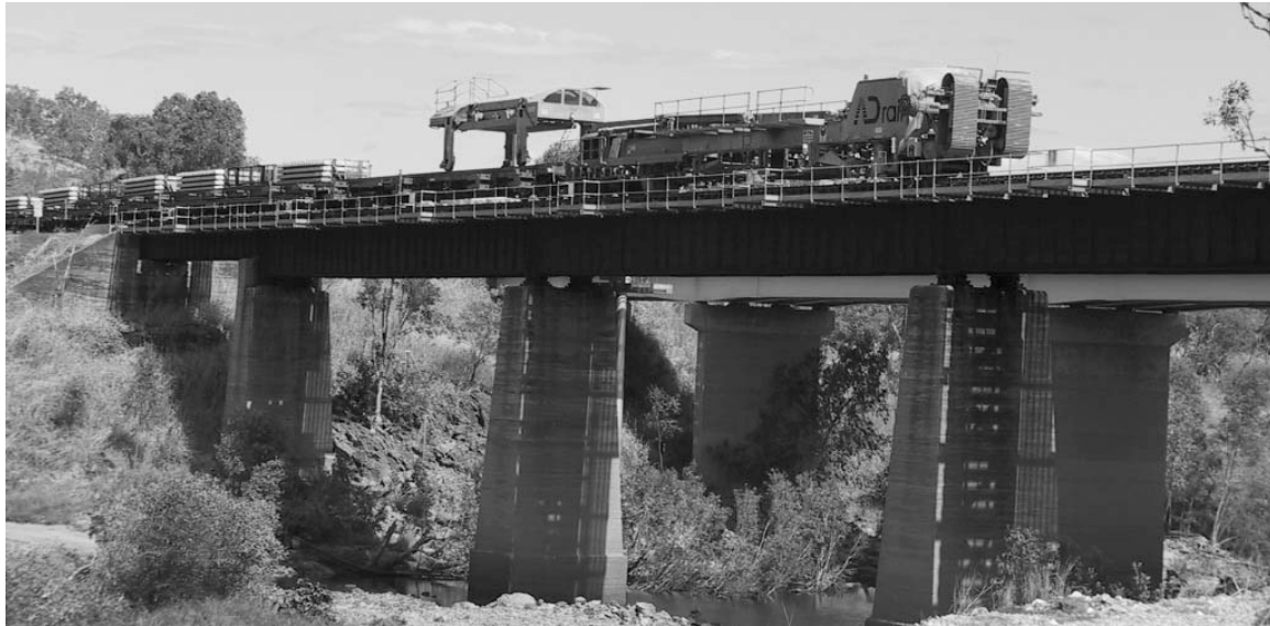
Figure 7 –Recycled Fergusson River Bridge
