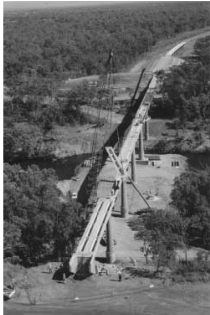
Figure 3 – Katherine River Bridge
