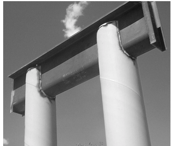
Figure 6 – Typical Minor Bridge Pier
