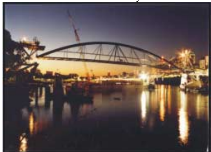
Figure 10: Main span lift
