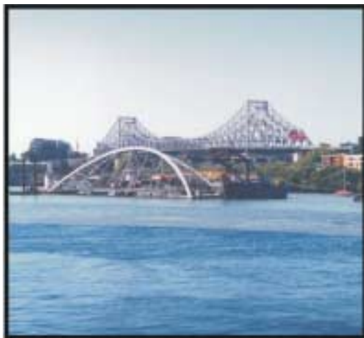
Figure 9: Main span on barge
