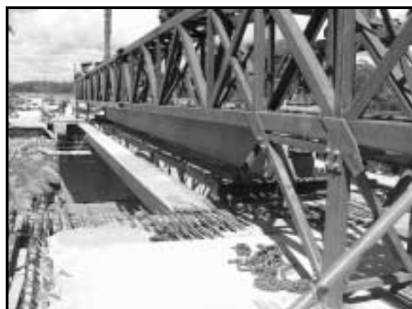
Figure 5: Launching Truss supporting Beam
