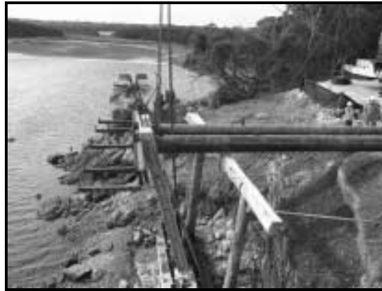
Figure 4: Temporary Support for Pier
