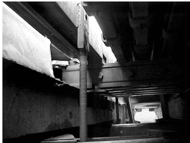
State of Pheasants Nest southbound bridge expansion joint before replacement
