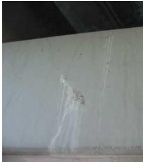
**Figure 10:** Close up of a shear crack in the crosshead.
