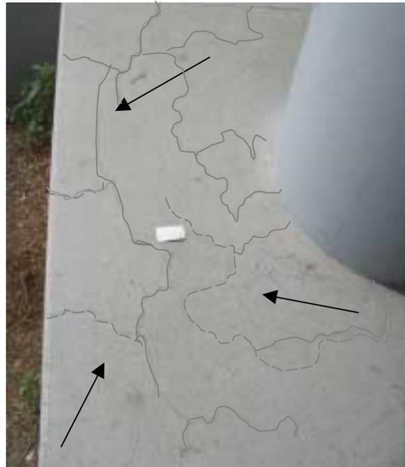
***Figure 12: Map-cracking in the north end of pile cap of Pier 1, probably due to drying-shrinkage.***
