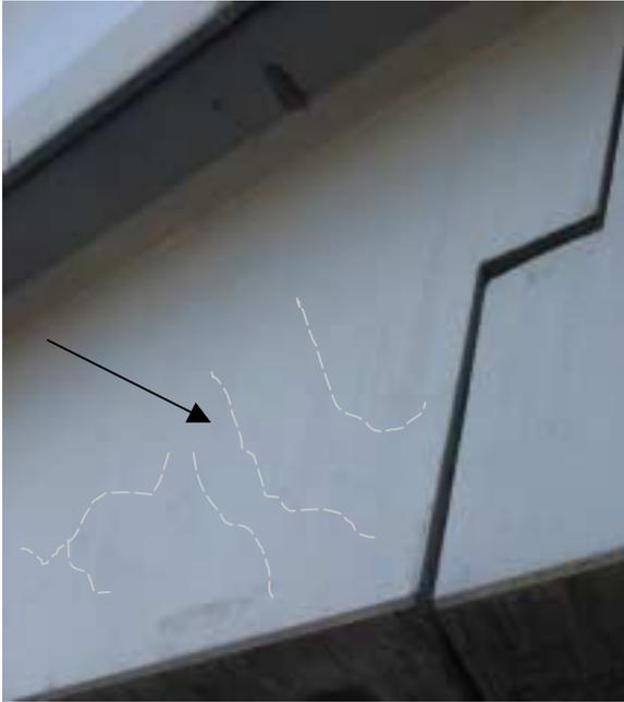
**Figure 7:** Weak radial cracking at the lower corner of the left beam (southernmost beam, middle span).
