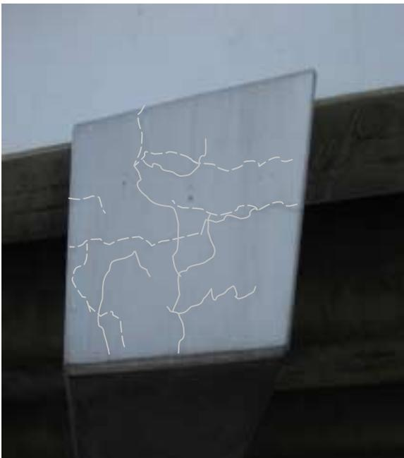
**Figure 9:** Map-cracking at the south end of the south bridge crosshead. Cracking extends into the element.
