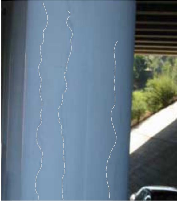
***Figure 11: Multiple parallel vertical cracking in the southern-most column of Pier 2.***
