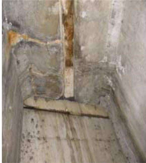
**Figure 8:** Cracking in the flange of some super T-Beams at the left abutment, probably resulting from mishandling or impact by heavy vehicles.
