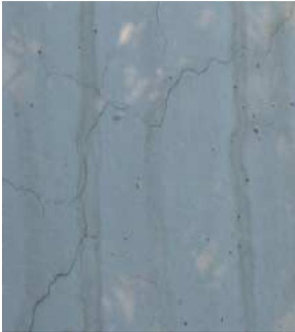
*Figure 5: Cracking in the north wall of the east abutment.*
