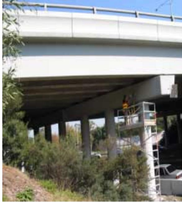
*Figure 1b: Pier 2 from which cores were taken, viewed from the North.*
