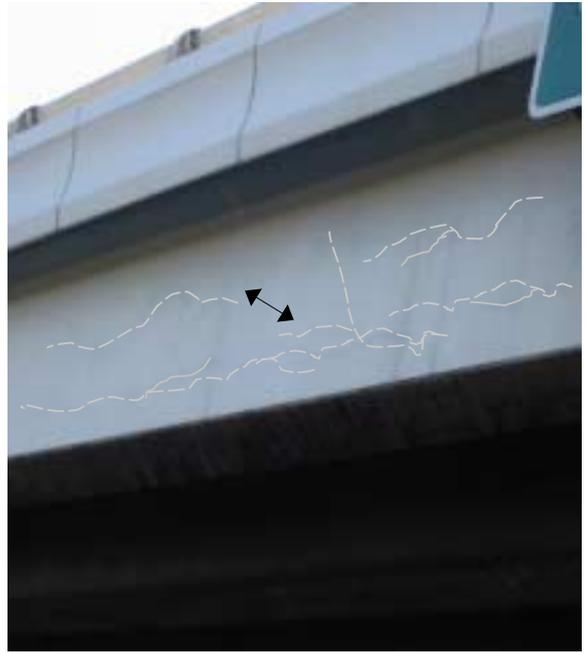
*Figure 6: Longitudinal parallel cracking on the exterior face of the southern-most beam of the middle span.*
