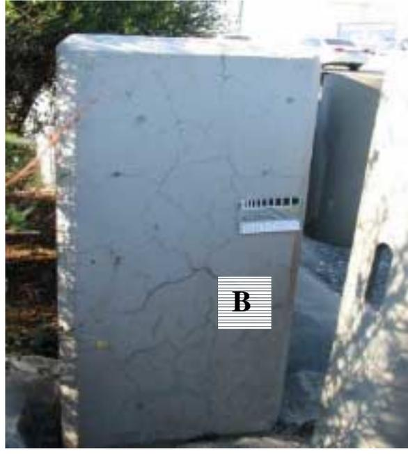
*Figure 4: Cracking in the base of the parapet unit (4A) and in a post (4B).*
