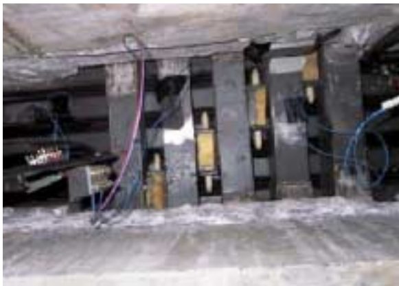
Figure 15: Experimental Modal Analysis of existing Multi Support arm Modular Joint at Taree.
