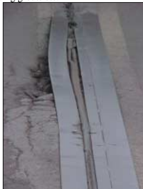
Figure 5: Often encountered failure of cast-in steel retainers. Fatigue of retention ligatures or concrete failure behind angles
