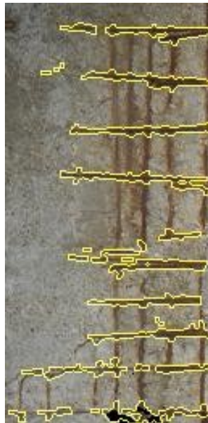
Horizontal reinforcement (stir-ups)
