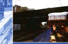
WEIGHT CONSCIOUS: To reduce the weight of the bridge the exciting surface was removed and replaced with a lightweight concrete.
