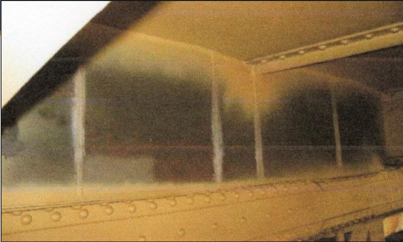
Diaphragm between main girder top boom and deck plates to transfer shear loads
