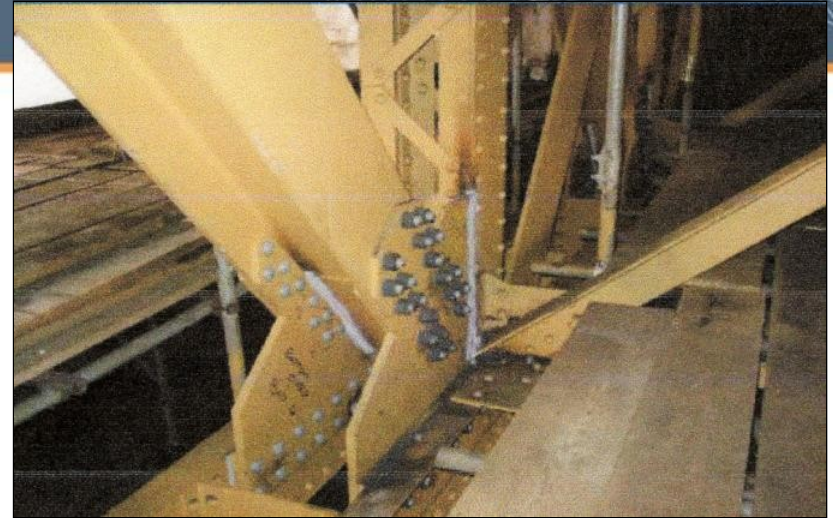
Strengthening of main truss ties with new "H" beams
