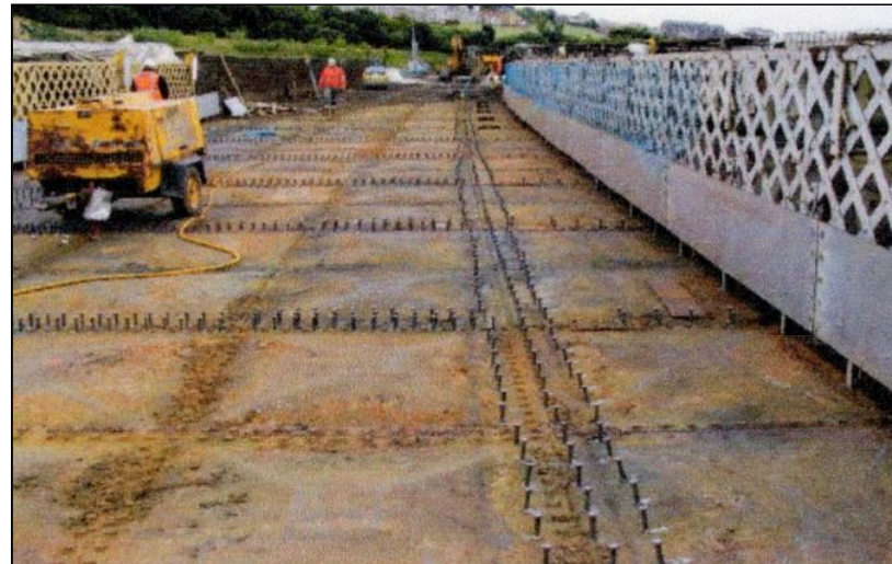
8,600 shear studs attached for new concrete deck
