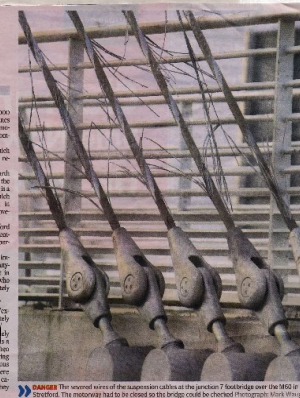
» DANGER The severed wires of the suspension cables at the junction 7 footbridge over the M63 in Stretford. The motorway had to be closed so the bridge could be checked. Photograph: Mark Wain
